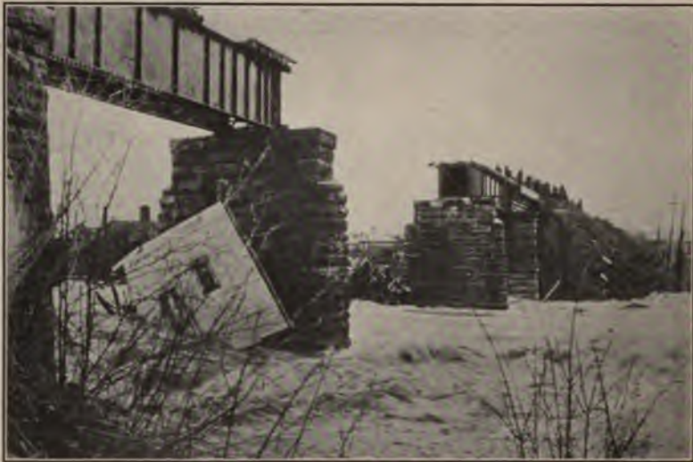
FIG. 17.—The flood passing the Big Four R. R. bridge at Delaware. The 1913 flood "headed up" nearly 5 ft. at this bridge, furnishing means for an approximate estimate of the flow.
